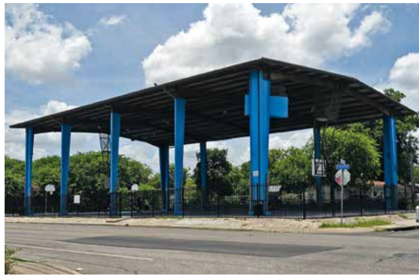
Fig. 5.8.6. The shade structure above this basketball court in San Antonio, Texas, USA, provides sun protection.
