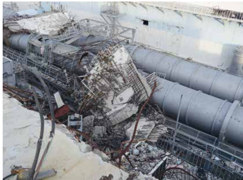
Fig. 2.5.3. Debris from the upper levels of unit 4 at the Fukushima Daiichi power plant in December 2012, 21 months after the nuclear accident.
