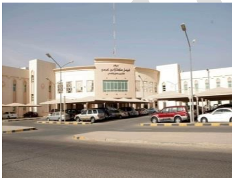
Faisal Sultan bin Essa Center for diagnostic and Radiation therapy
